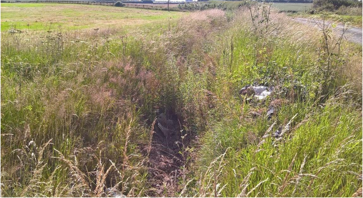
Image A1.1: Dry vegetated ditch.
